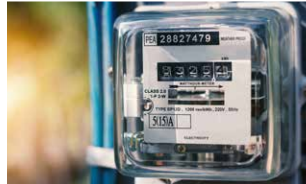
LEVEL 2: RELOCATE UTILITIES
